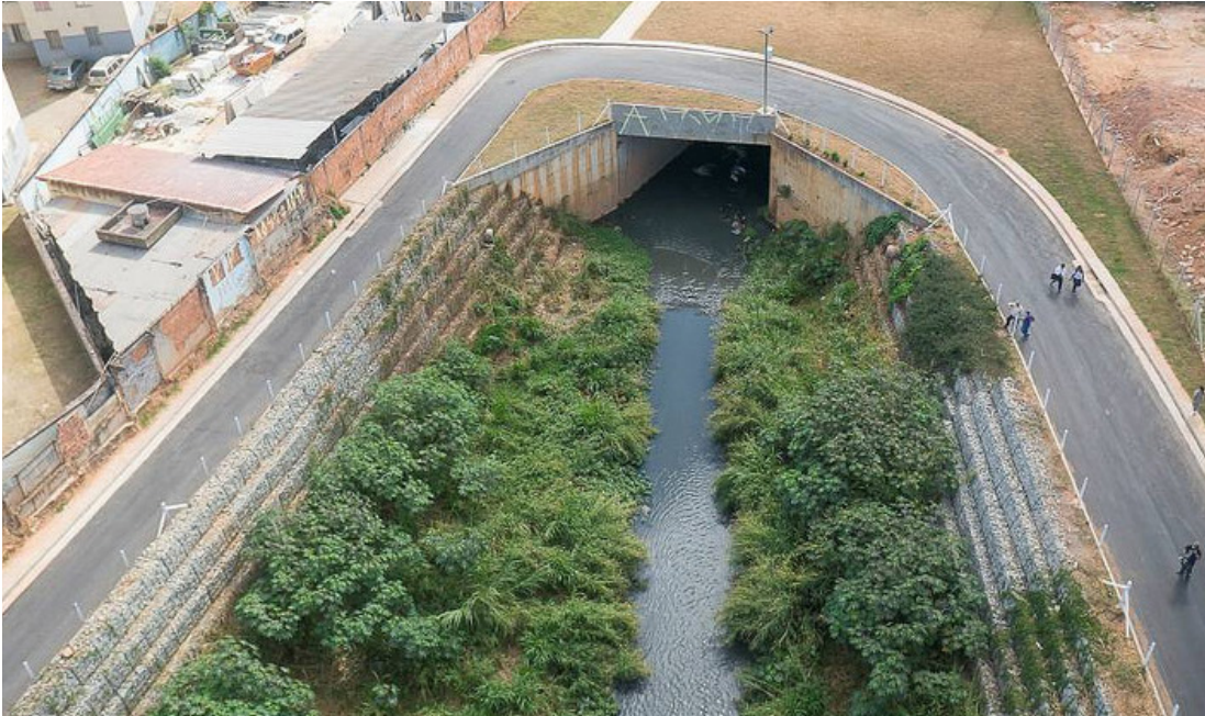
Figure 10.3: An example of channelisation which provides formal constraints to contain flood waters
