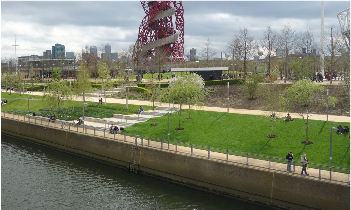
Figure 10.5: An example of a linear park designed with embankments that can flood (London, UK)
